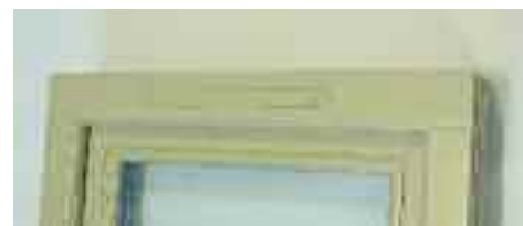
TRICKLE VENT DETAIL
